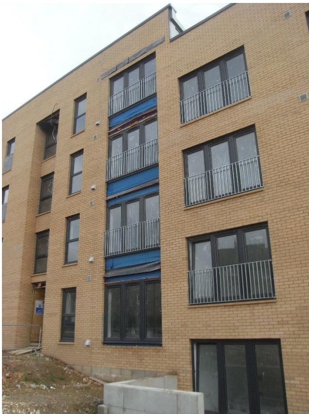
Block 5 – Window, facing brick, and Juliette balcony installation (28.09. 2021)
