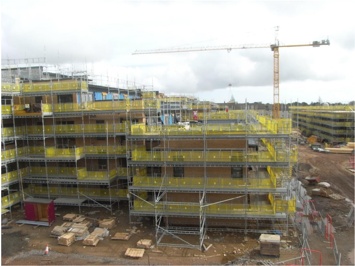
Foreground – Block 2; Background right – Block 6 (28.09.2021)
