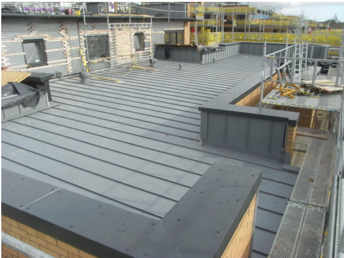
Block 1 – Vico Roofing complete; Corium cladding in progress (28.09.2021)
