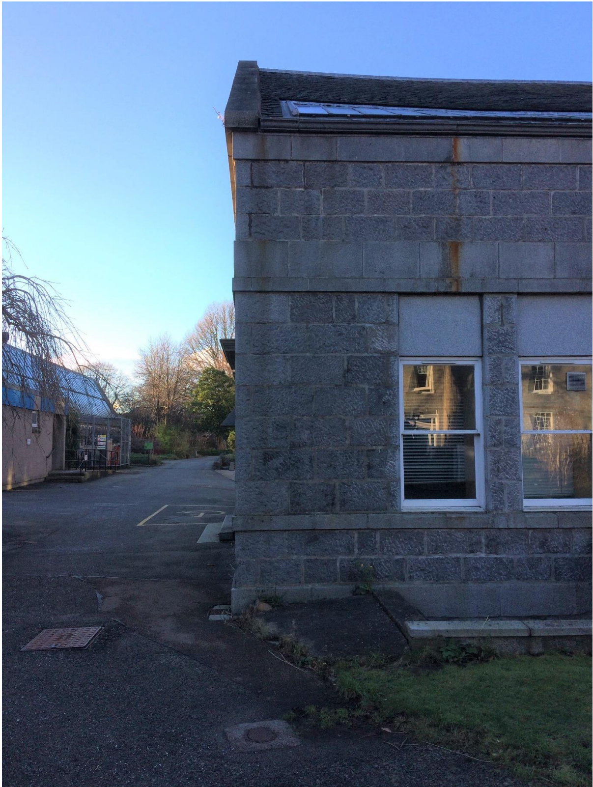
Appendix 2: Photograph of Proposed Location on Cruikshank Building.
