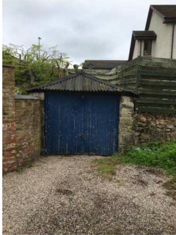
GARAGE SOUTH WALL
