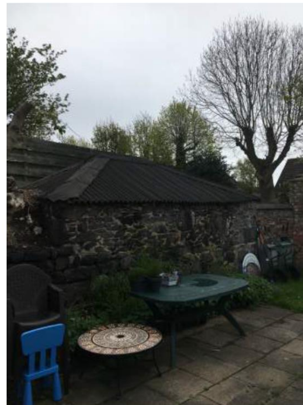
GARAGE WEST WALL
