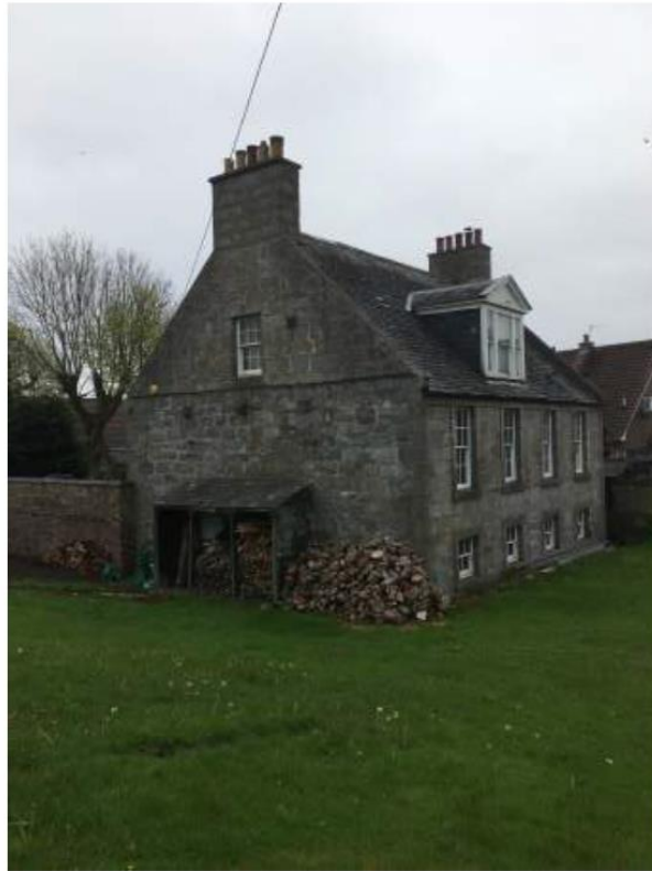
NORTH / WEST WALLS
