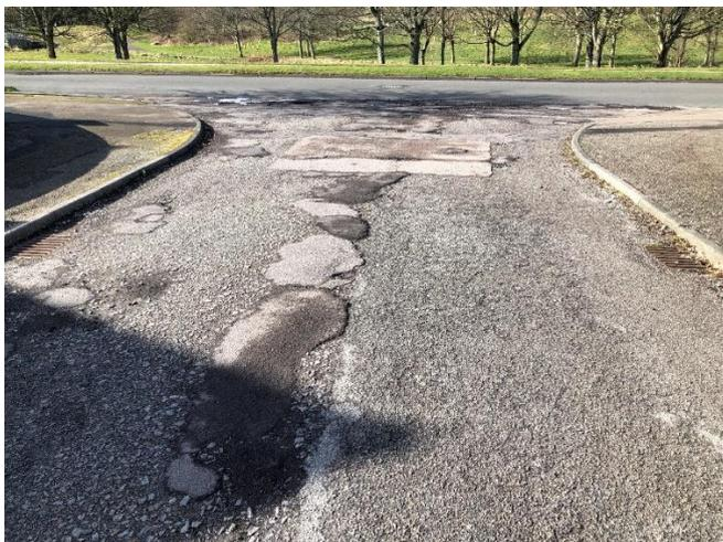
Stronsay Avenue junction with Stronsay Drive; Severe deterioration with multiple repairs.
