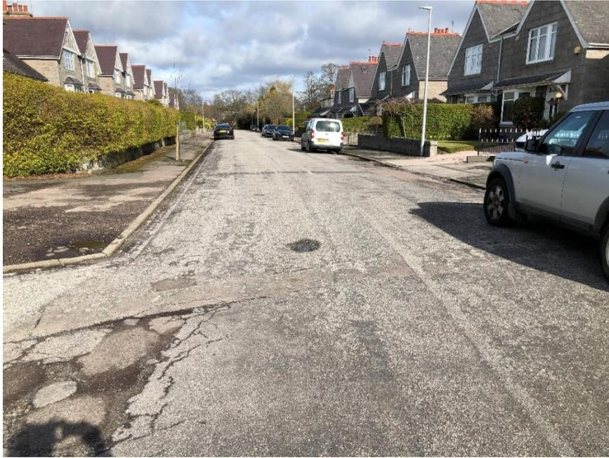
Northburn Avenue is in generally fair condition. Whilst worn, it is free of any significant defects and shows no signs of significant deterioration. The surface appears stable and generally intact. Several localised areas of deterioration present. The road is in good, serviceable condition.
