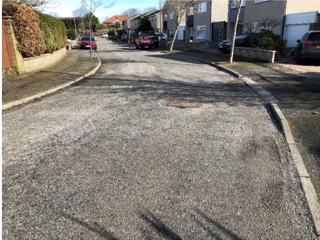
General condition of Stronsay Avenue. Significantly worn, but serviceable and largely free of major defects. The surface is typical of streets of this age. The condition does not present danger to road users and is unlikely to suffer significant and rapid failure.
