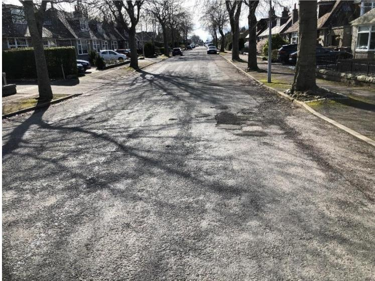
The general overall condition of Angusfield Avenue is worn, but serviceable with some larger areas of deterioration, and some areas of recurring potholing.
