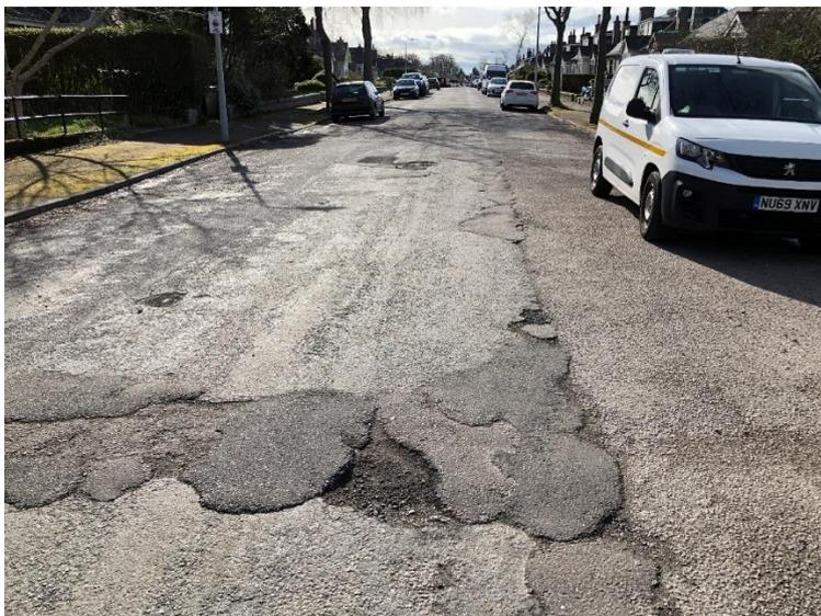
General deterioration in areas of Angusfield Avenue. Multiple utility tracks failing which require remedial works.
