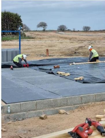
**Photo 1 – Membrane works underway at the initial flatted blocks**
