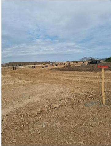
**Photo 5 – Road formation with foul and surface manhole cylinders visible in the distance**
