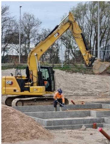
**Photo 3 – Underbuilding platform being smoothed for installation of DPM and insulation**
