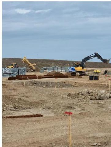
**Photo 4 – Structural fill platforms being upfilled**
