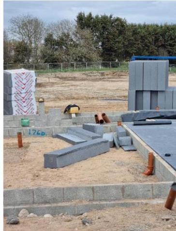
**Photo 2 – Blocks of insulation being installed at the initial flatted blocks**
