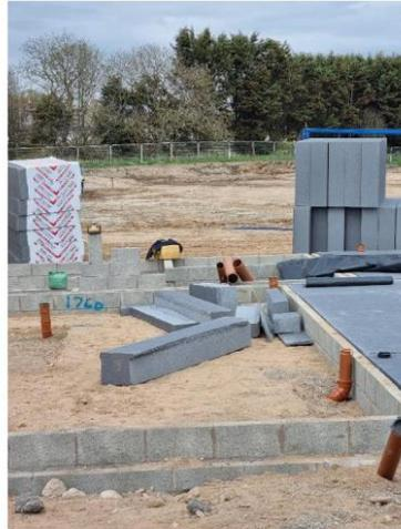
**Photo 2 – Blocks of insulation being installed at the initial flatted blocks**
