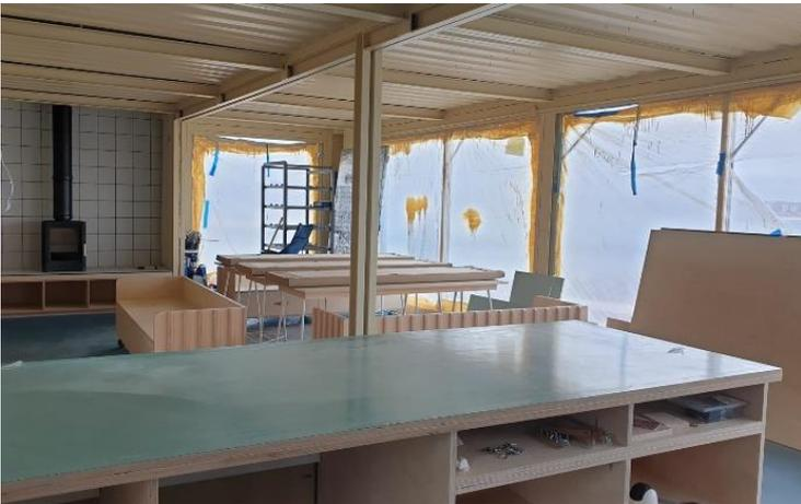
Works included the installation of walkways and decking, cladding, and roofing, internal joinery and bespoke furniture and fit of the kitchen.
