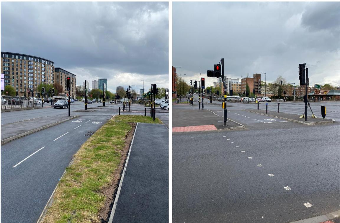
Figure 4.2: Two-way segregated cycle track – Examples
