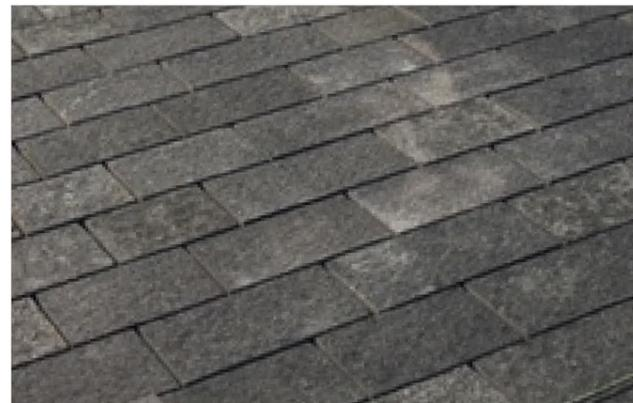
Lay-bys / pedestrian thresholds / vehicular overrun on pavements - Dark Whinstone Setts
