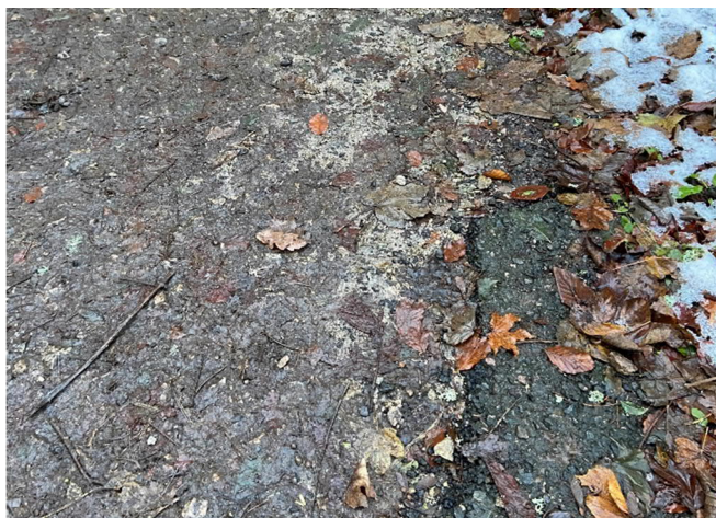
Figure E.2: Surfacing west of Glebe Park
