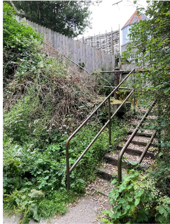
Figure 5.18: Deeside Way Access at Westerton Road
