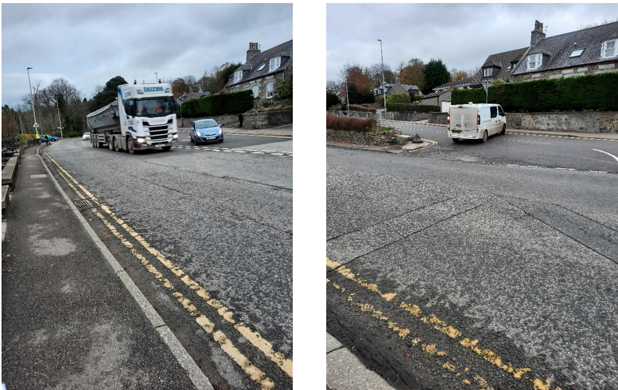
Figure D.4: Safety Concerns at the A93 / Malcolm Road (B979) Junction
