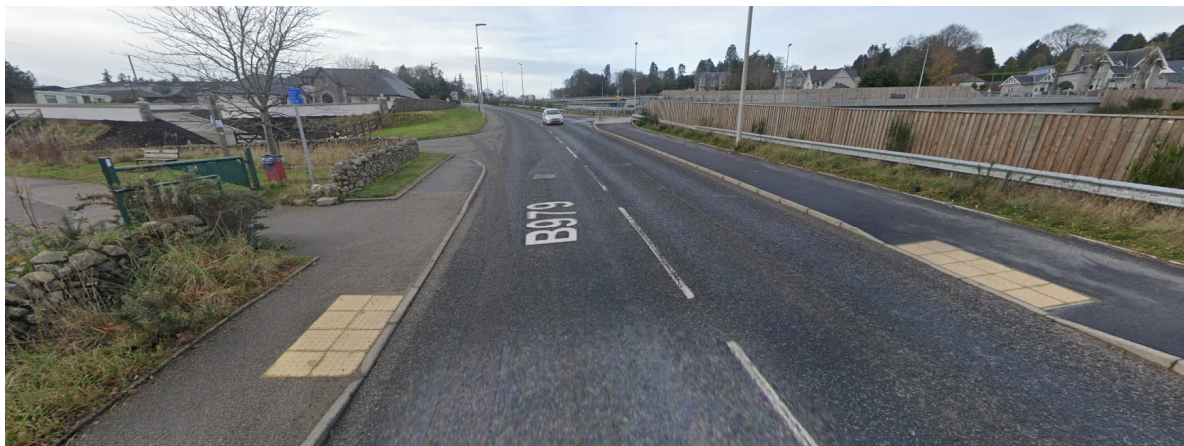
Figure 5.30: Existing Crossing on B979 connecting Deeside Way (Source: Google Street View)
