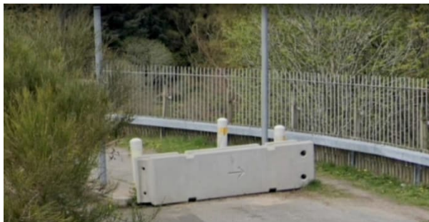
Figure 5.54: Park Bridge Access Controls
