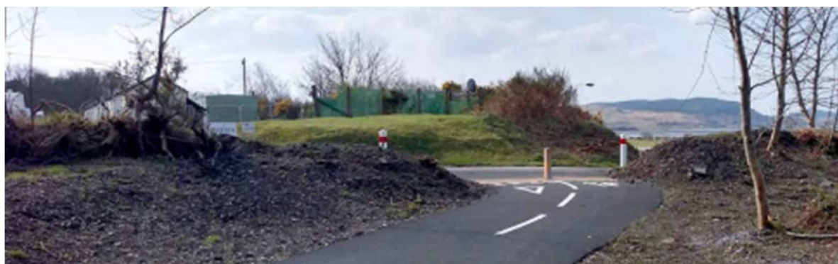
Figure 5.6: Bollard Access Control Example
