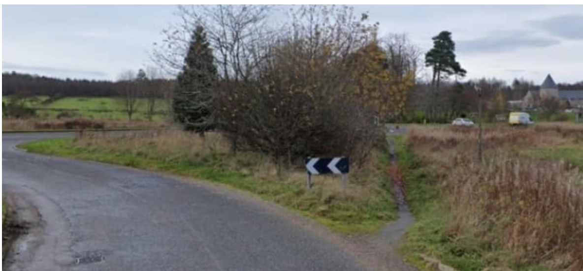
Figure 5.22: Desire Line to A93 (Source: Google Street View)
