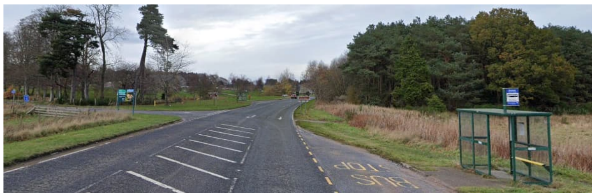
Figure 5.32: A93 at Drum Castle Junction - Existing Provision (Source: Google Street View)
