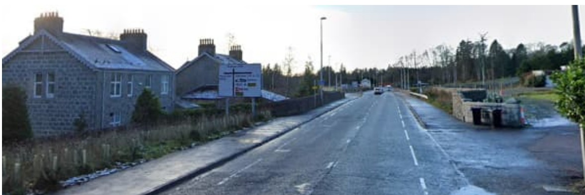
Figure 5.29: Bellenden Walk/A93 Junction - Existing Provision (Source: Google Street View)
