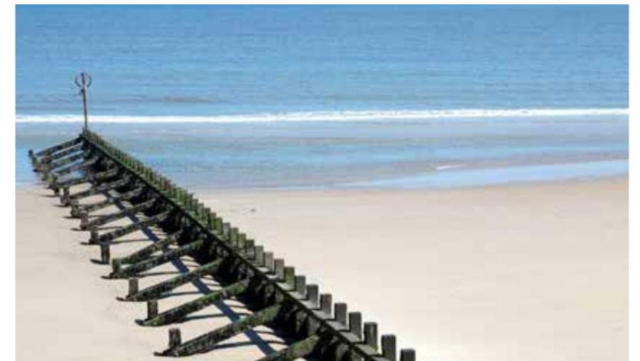
Image of the groyne structures which are positioned along Aberdeen Beach
