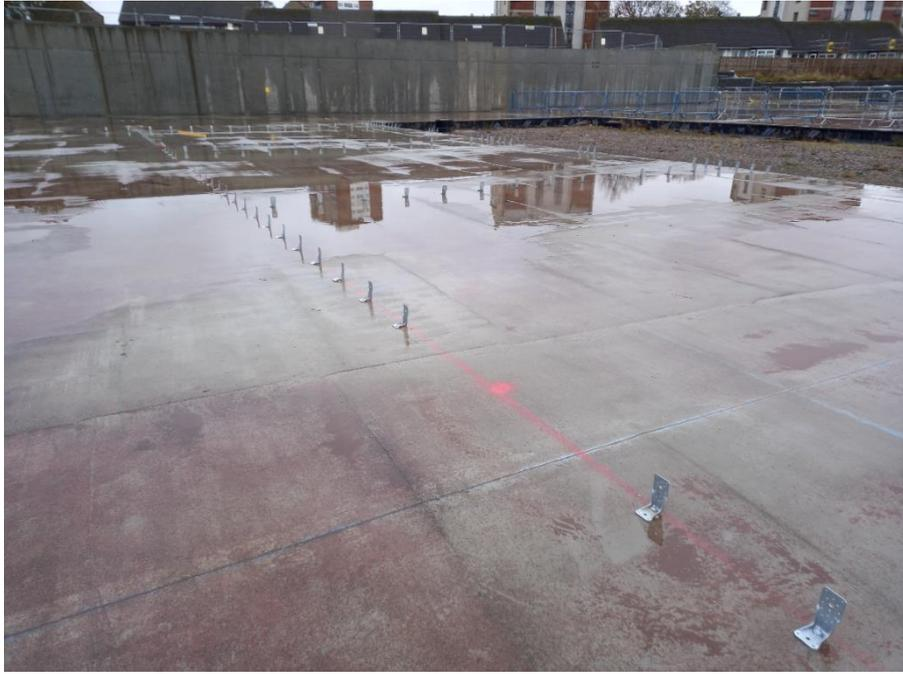
Brackets installed on lower ground floor slab ahead of cross laminated structure
