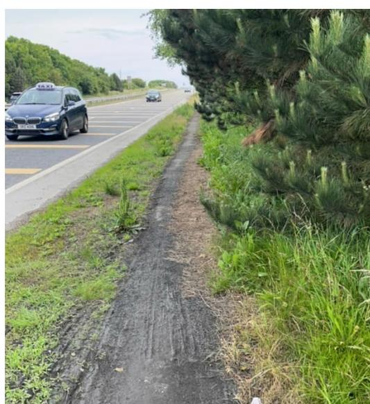
Figure 2 Existing Footway Condition - Overgrown Vegetation
